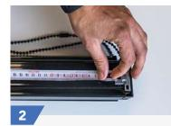
**Take your measurements:** plan the holes at 10 / 15 cm from the ends of the fixing bar.
