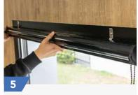
Once you have screwed in your 2 fixings, you simply clip on the film blind fixing bar directly.
